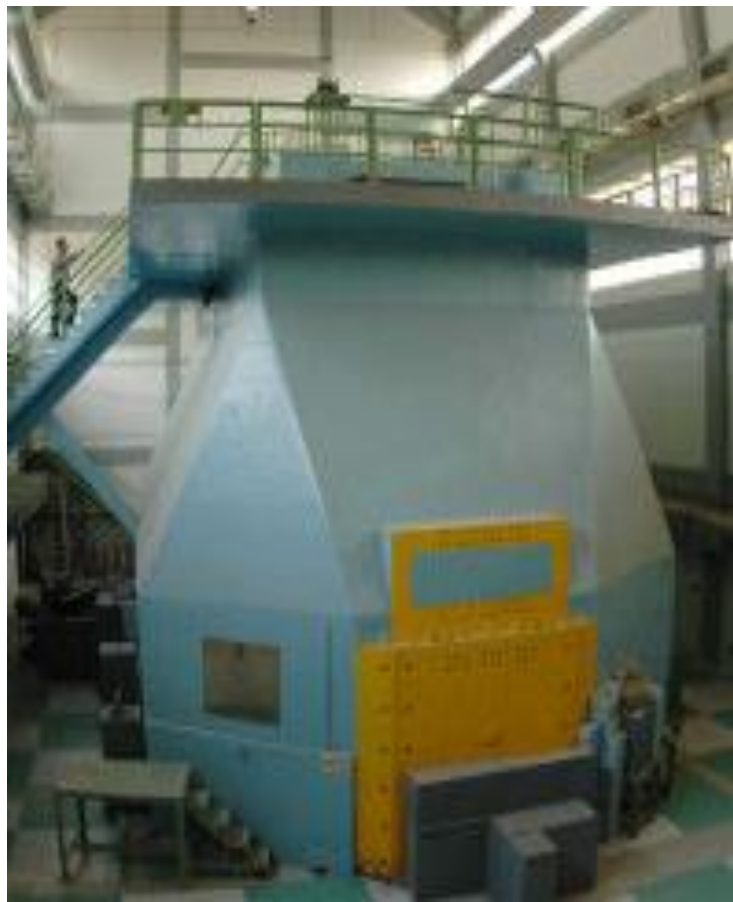
Apsara Research Reactor
